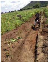
Excavation of land for the ongoing fencing of the One-hectare plot for ESN National Secretariat in Abuja
